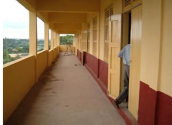
The Completed School Block
